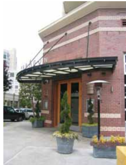
An attractive corner entry creates a more inviting public space at the corner.
