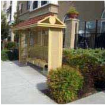
A landscaped setback provides privacy for residents and space for transit stop amenities.
