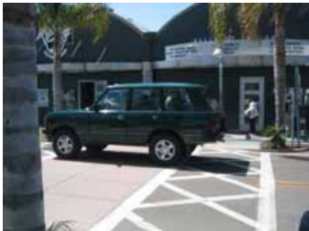
A raised crossing causes vehicles to have to slow and eases pedestrian crossing.
